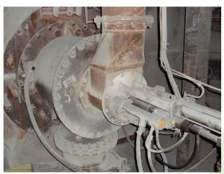
1. Installation for coal ignition in heat and power generating plants
